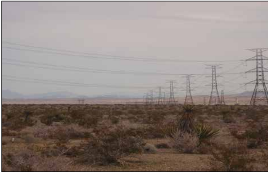
View from KOP #1 – looking North
