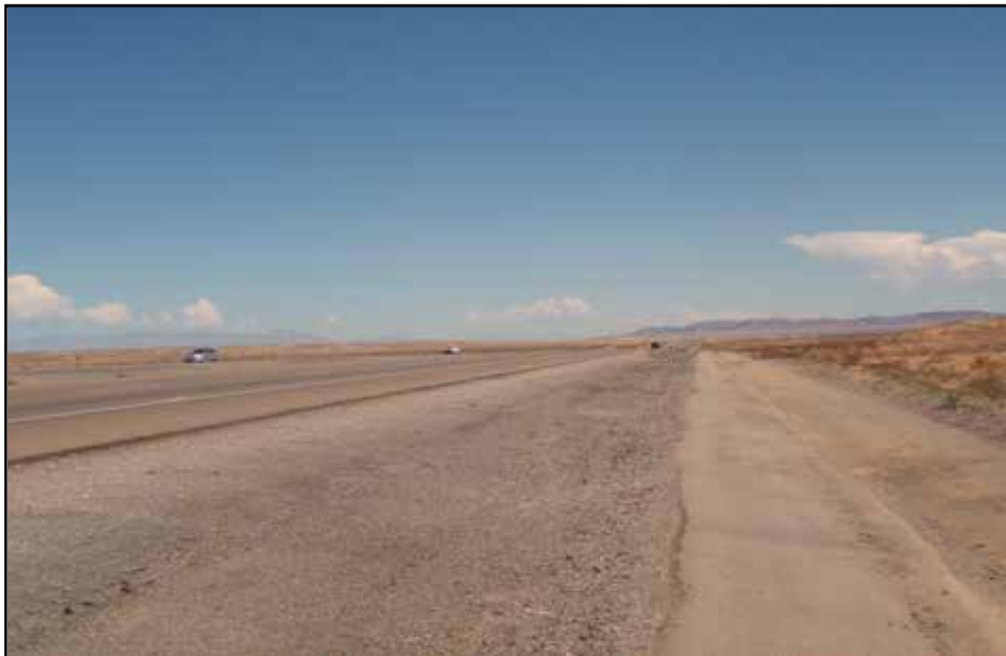
View from KOP #3 – looking North
